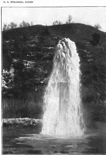
U. S. GEOLOGICAL SURVEY 4. ARTESIAN WELL AT LYNCH, NEBR. Flows more than 3,000 gallons per minute.
